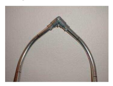
Slip the pull elbow over the ends of the conduit and tighten down the screws. Make sure the conduit goes all the way in. If it doesn't fit quite right, go back and fine-tune your bends.
